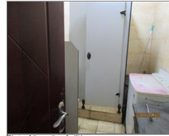
Photo of the sanitary facilities Toilet.JPG
